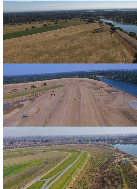
Southport Levee, West Sacramento
